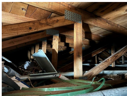
View of Wood Truss System
