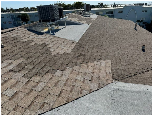
General View of Rooftop
