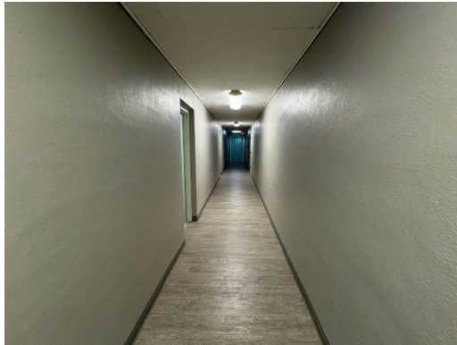
View of Typical Interior Hallway
