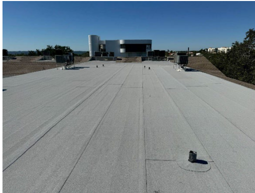
General View of Rooftop
