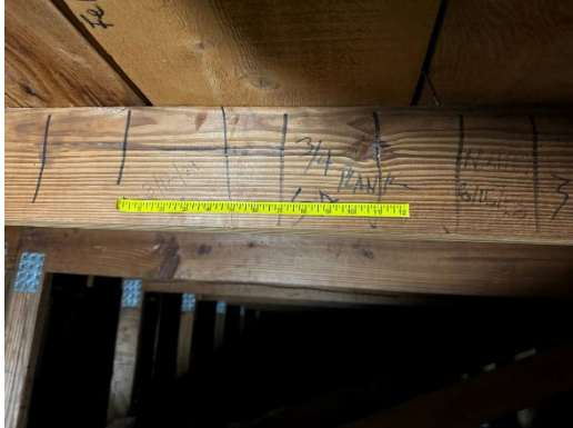
View of Roof Sheathing Nailing Pattern
